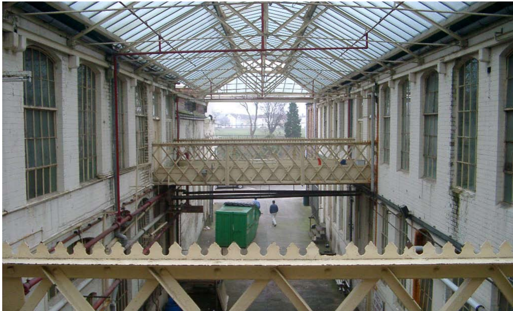
Left Present day view inside one of the covered haulingways
